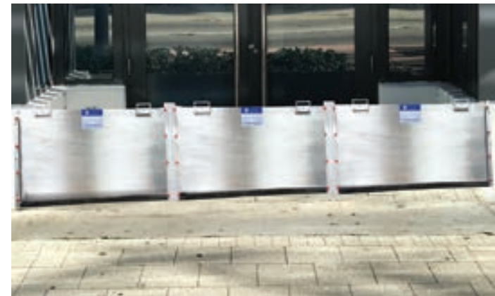
#5129MA mounted to front of hotel entrance.
