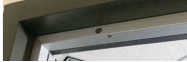
#5077CA Installed on head of frame.
